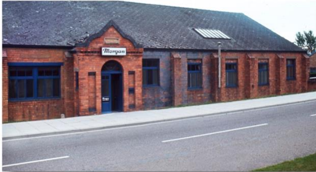
Front and side view of the morgan factory
